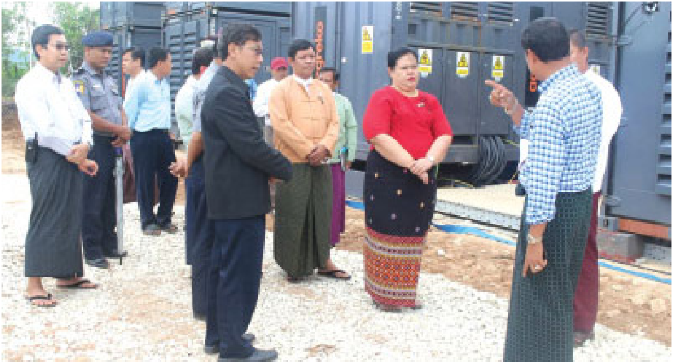
The Chief Minister of Tanintharyi Region government and the Minister of Electricity visit the electricity production site of GGS in Kanpauk region in 2017. (Photo: Tanintharyi Region/fb)
